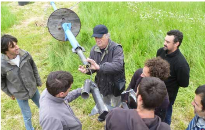
Fig. 19: Installing the alternator & frame
