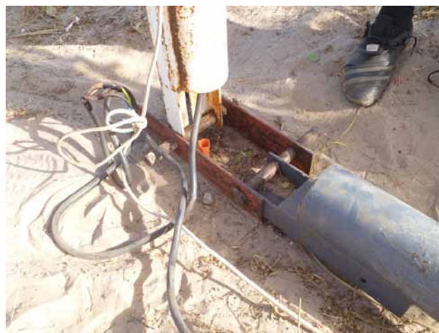
Fig 3: Sand at the tower base
