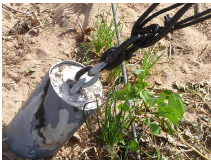
Fig. 5: Chain poured into concrete
