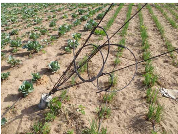
Fig. 4: Guy wires protected by oil
