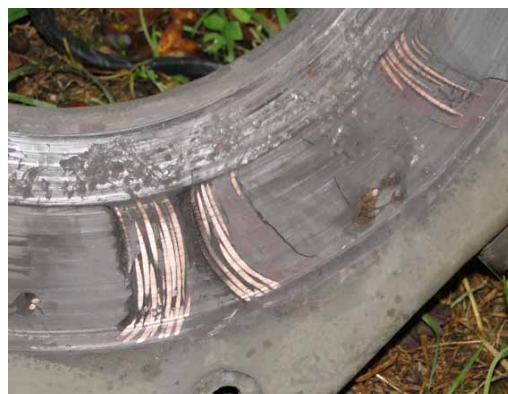
Fig. 34: Stator that needs to be changed
