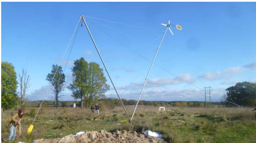
Fig. 15: Lowering the tower
