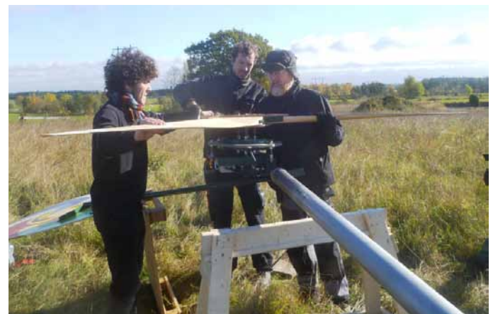
Fig. 21: Installing the blades
