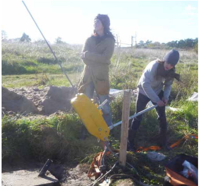
Fig. 23: Grip hoist to raise the tower
