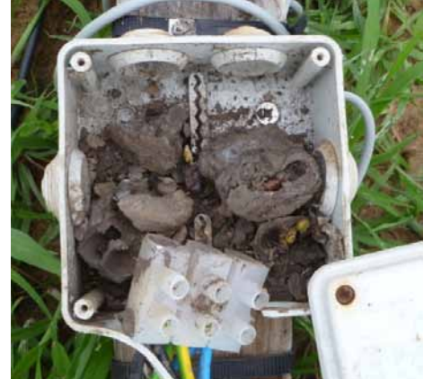
Fig. 48: Inhabitants in a junction box
