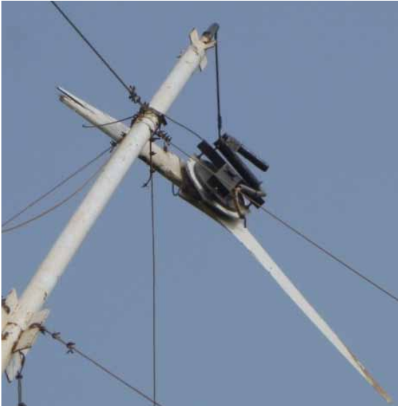
Fig. 42: Fall avoid by tight terminal block
